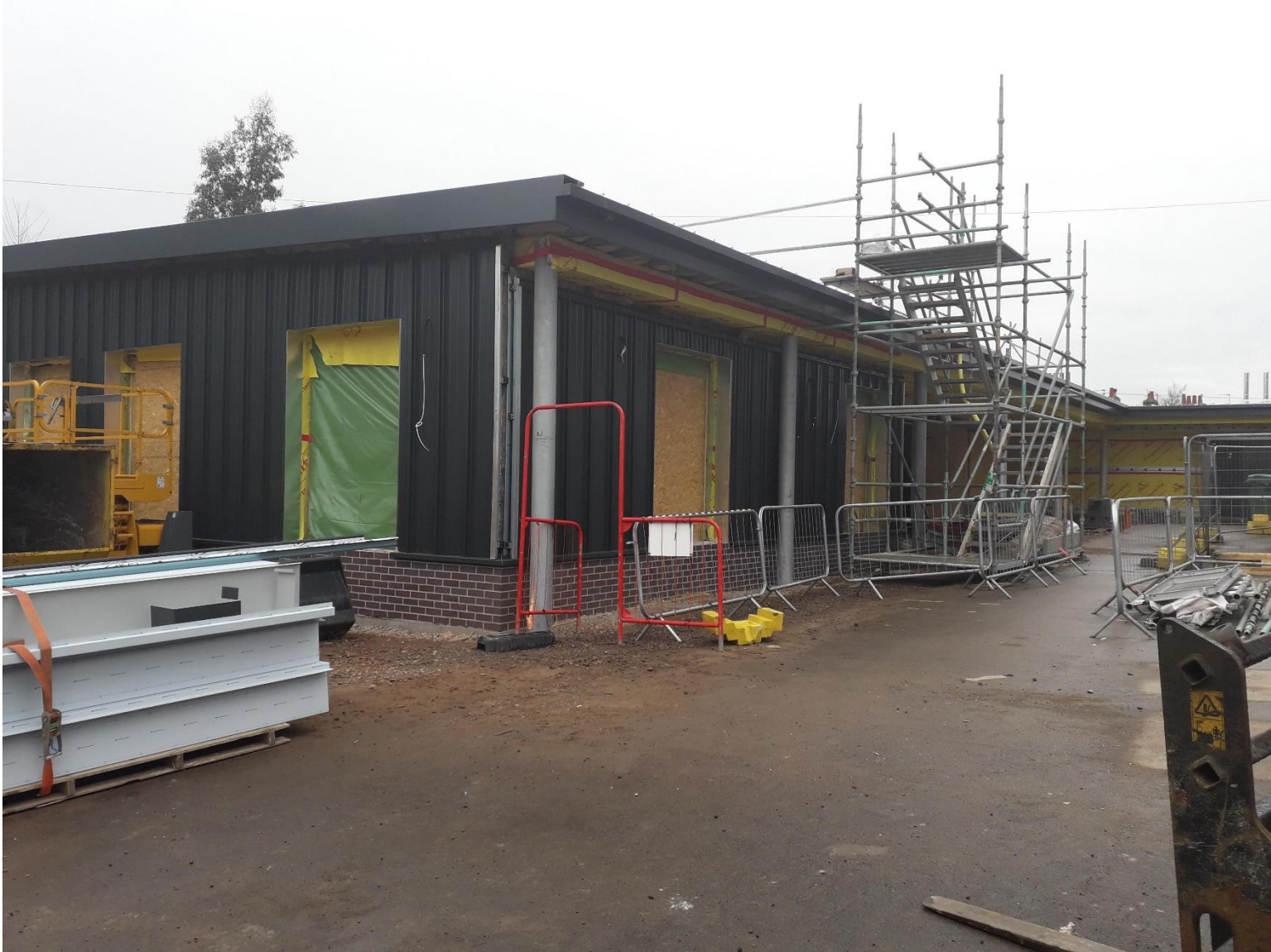
Broomhill – Progress Picture
