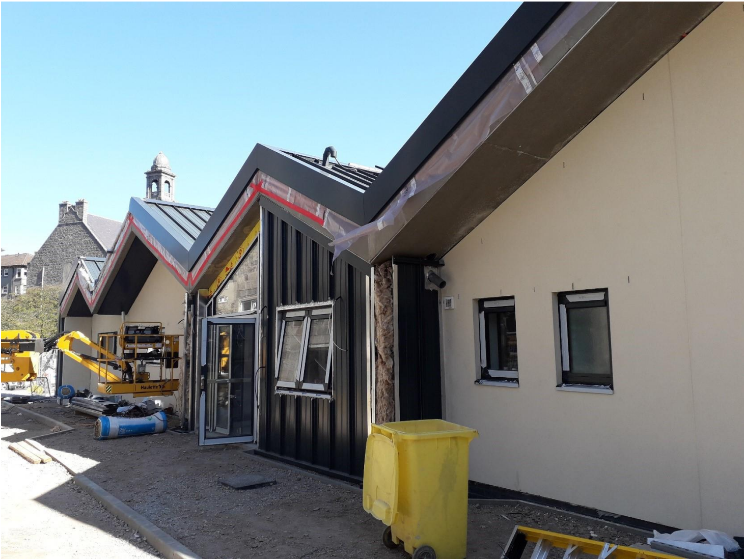
Gilcomstoun – Nearing Completion
