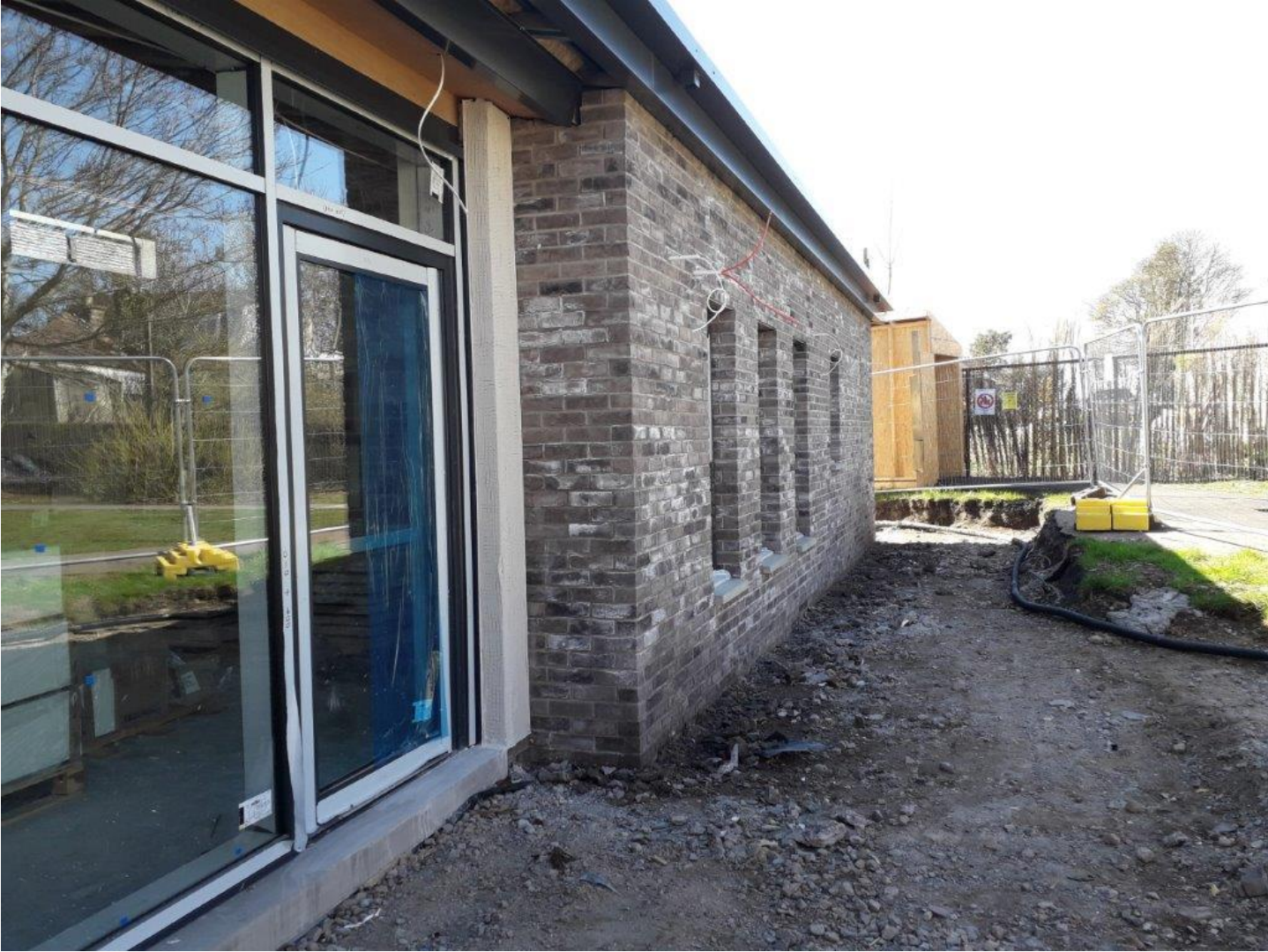
Culter – Nearing Completion
