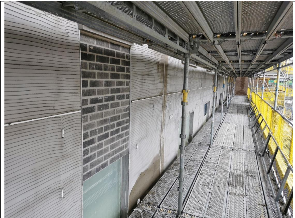
Block 2 Render Basecoat to West Elevation
