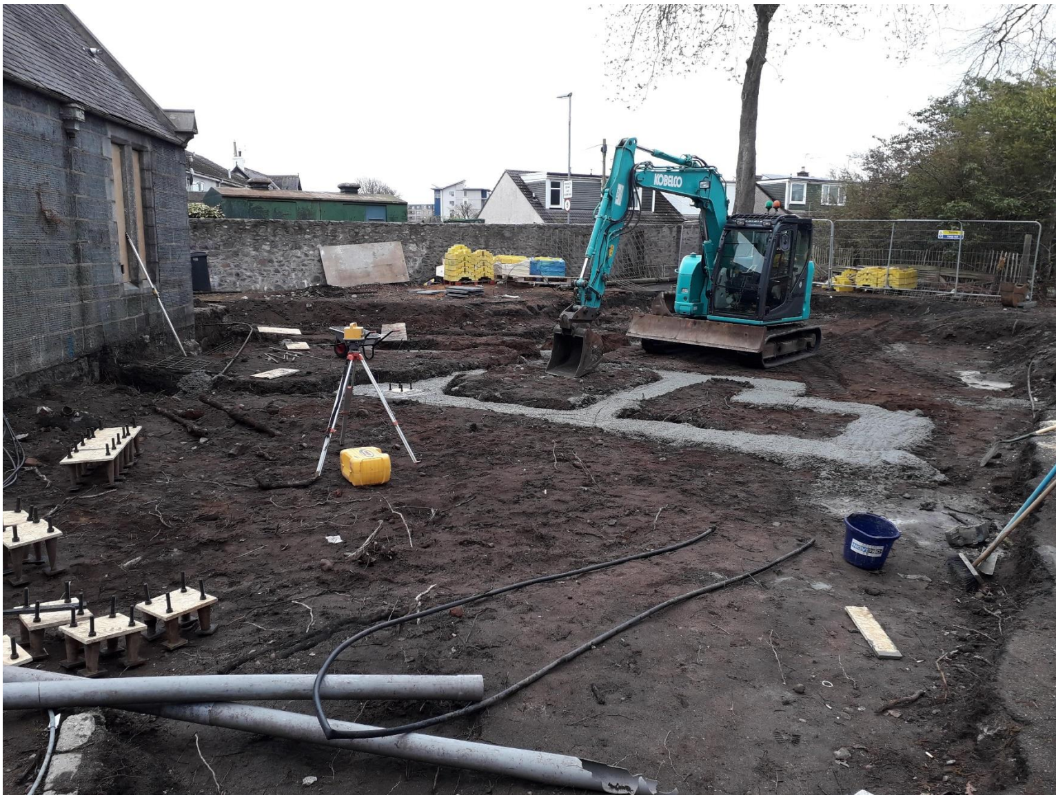
Duthie Park – Progress Picture
