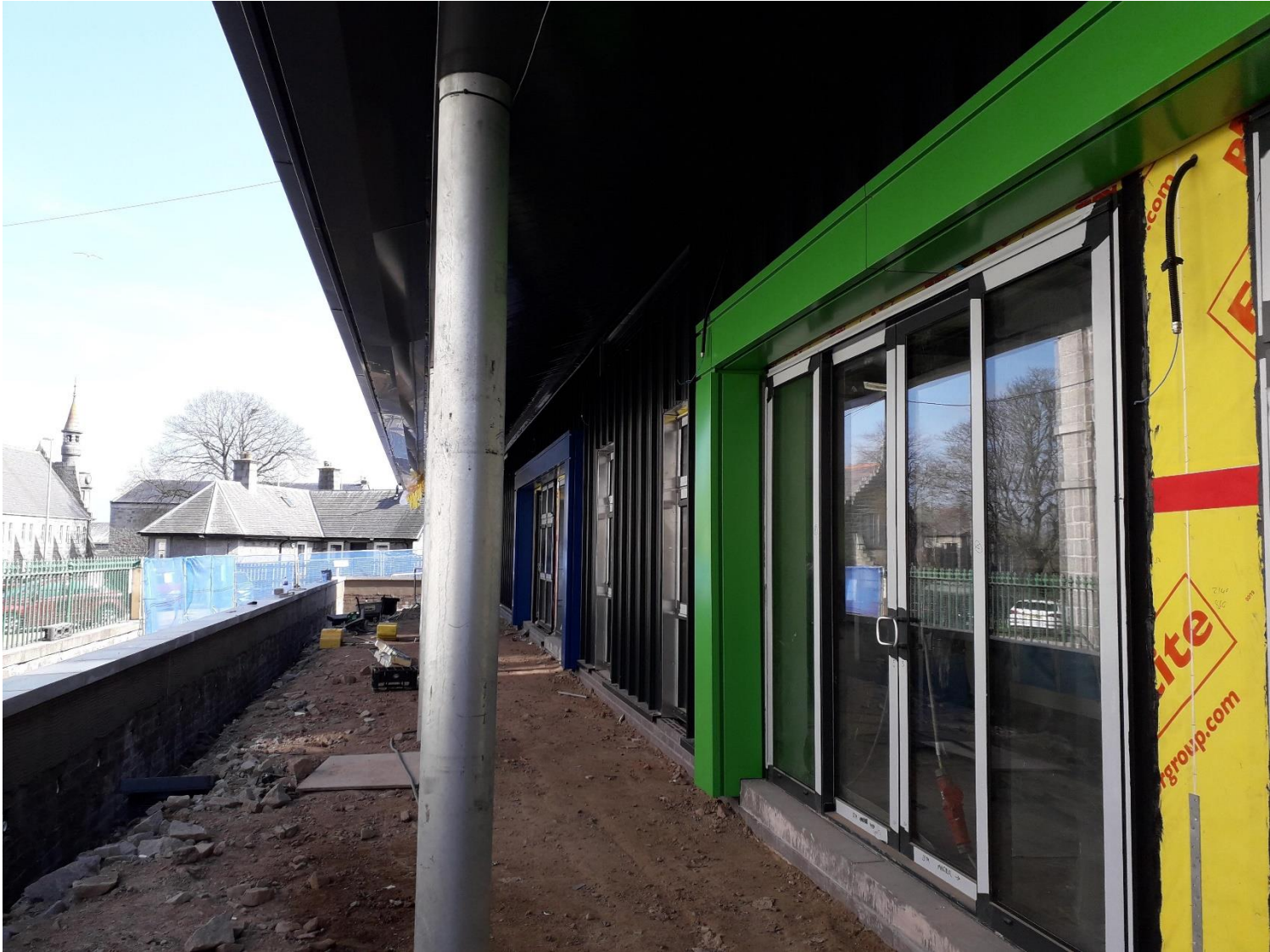
Woodside – Nearing Completion
