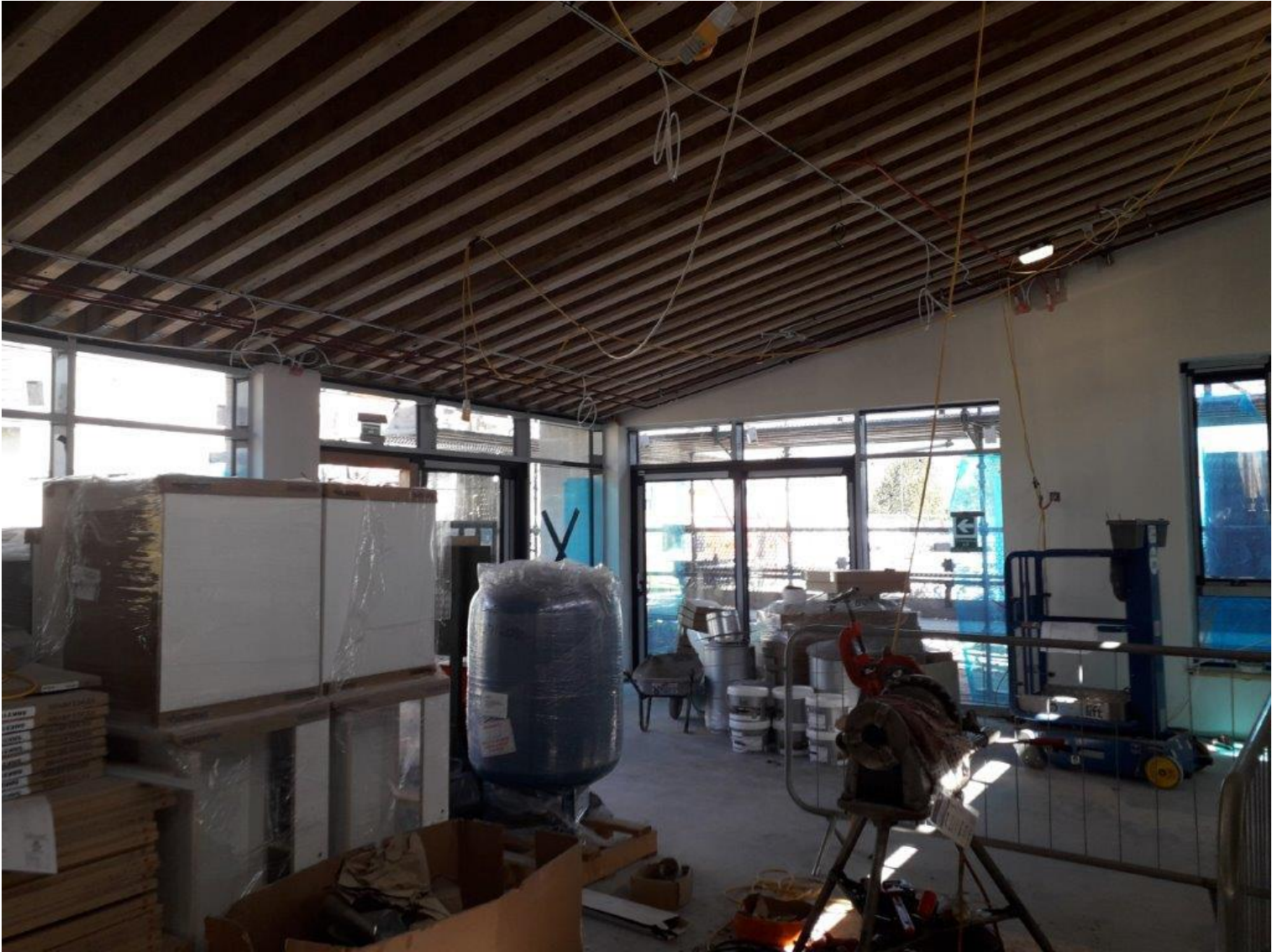
Culter – Nearing Completion
